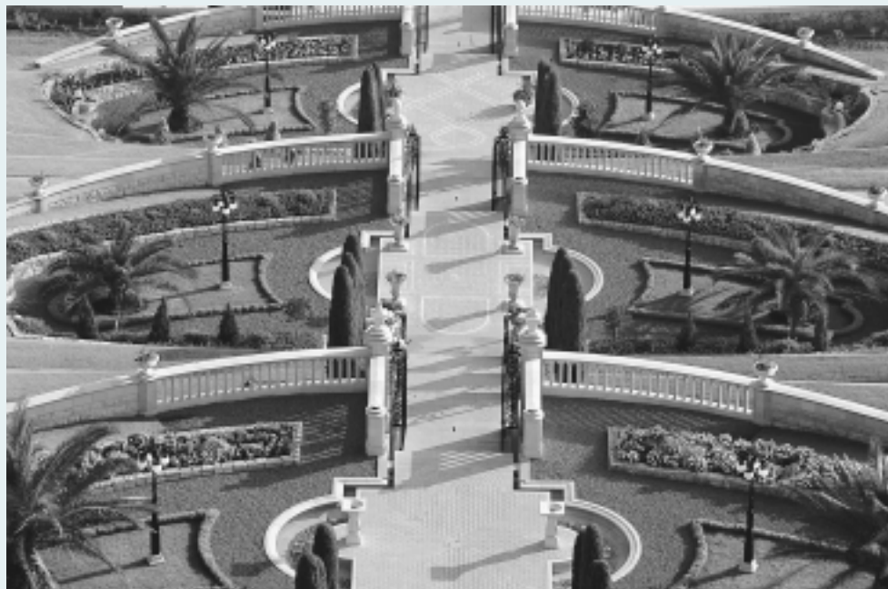
With a central stairway built of natural stone, and adorned with iron fixtures and marble fountains, the terraces on Mount Carmel have become a major tourist attraction in Israel.
