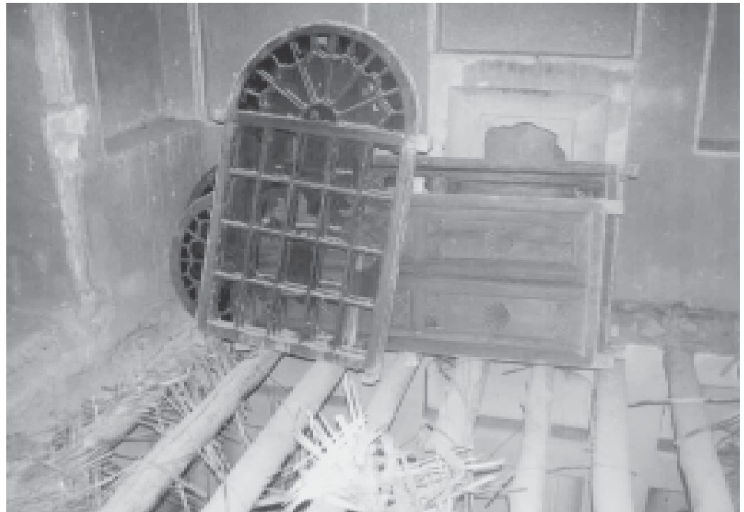
Even during its demolition by the Iranian government last June, the distinctive architectural features of the house of Mirza Abbas Nuri – a cultural landmark – are strikingly evident.
